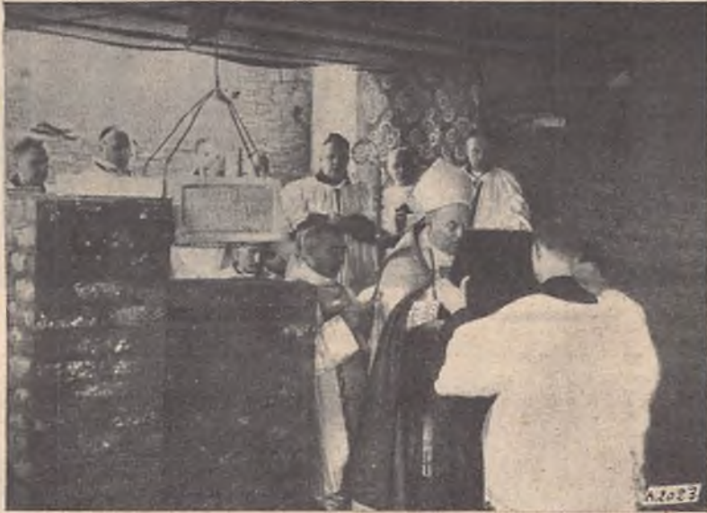
Laying the foundation stone for the church of the Belgian Salesian Theologate.
