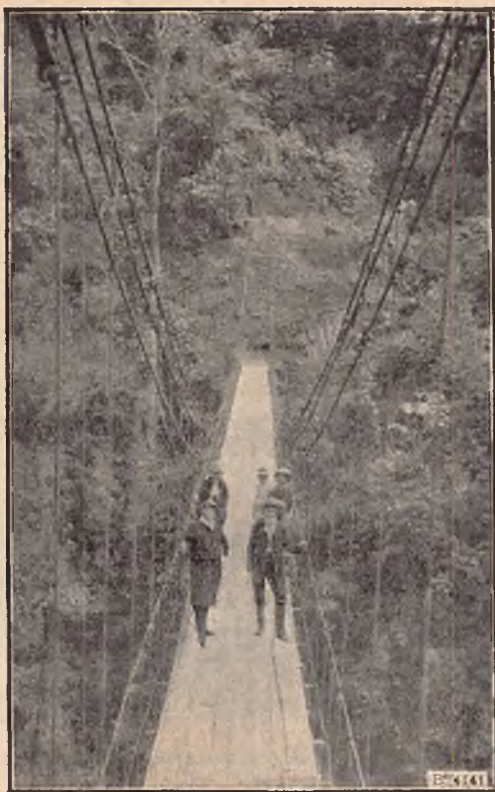
View of the new bridge from above the River.
