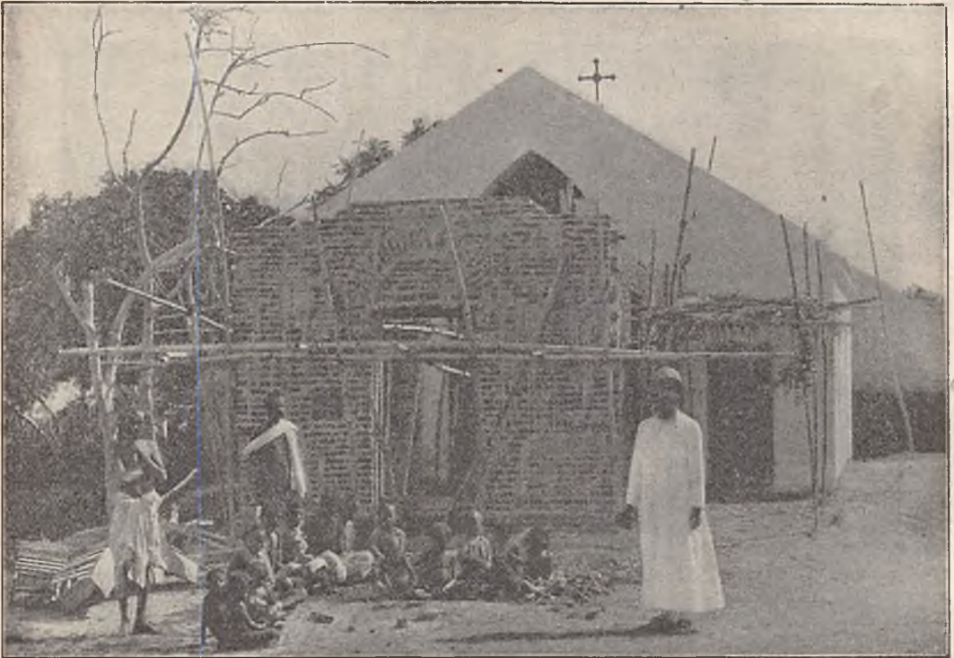
A New Salesian Church under Construction at Tanjore, India.
