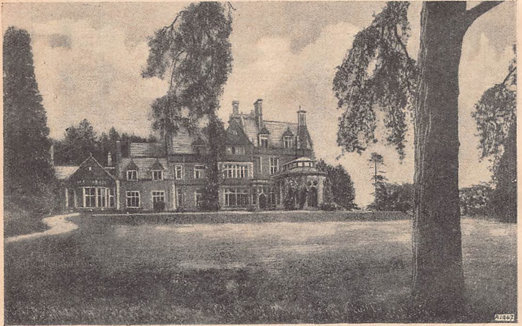
The new foundation in England of 1935.
