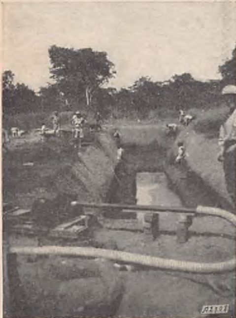
Belgian Congo. - Salesian missionaries constructing a canal.
