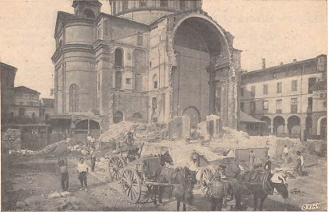
Demolition work goes on at the Basilica.
