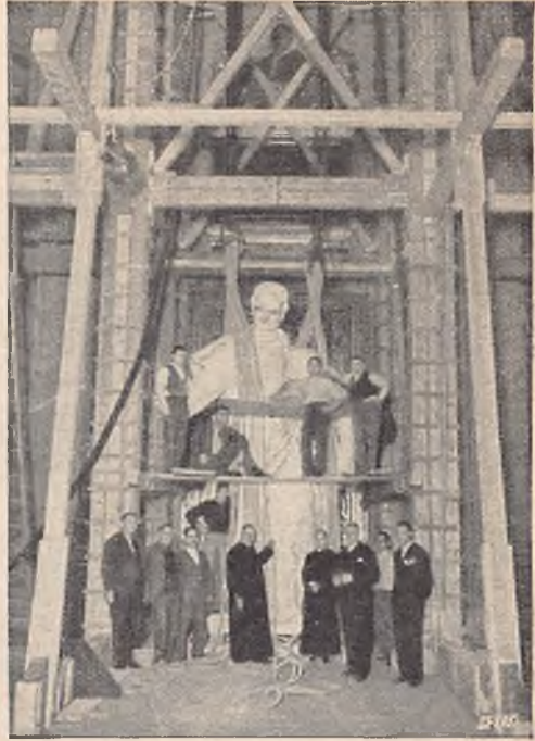
The statue group ready for hoisting into position.
