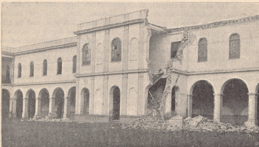
The western side of the Salesian Institute after the earthquake.
