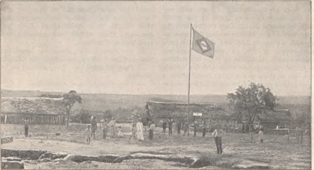
Sacred Heart Colony (Matto Grosso) - Central buildings, temporary chapel, etc.
