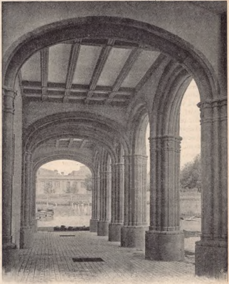
New Salesian House in course of construction in Lisbon.
