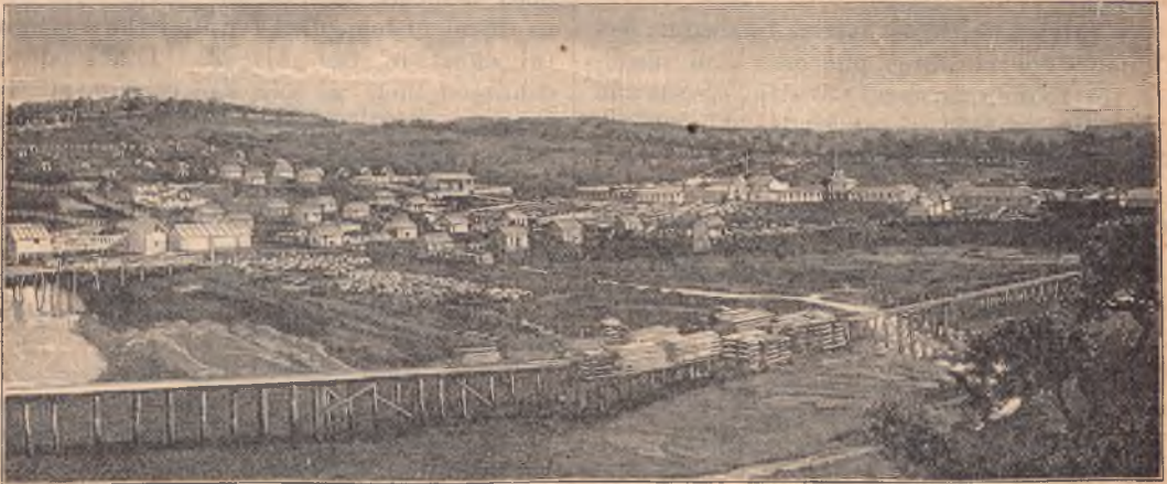
View of the Village constructed by our Missionaries on Dawson Island.
