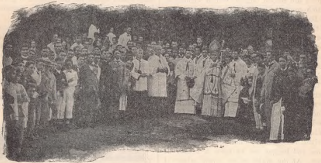
Laying foundation-stone of Church of Mary Ausiliatrice—Valencia.
